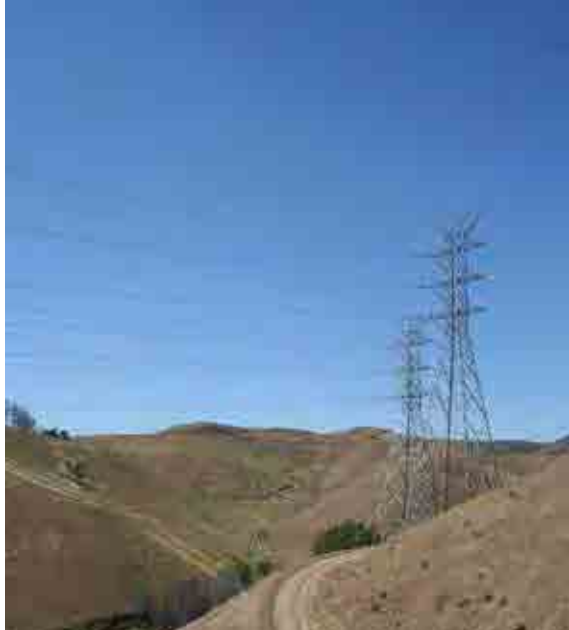
VISTA PARK CONNECTION TO PINE RIDGE FIRE ROAD
